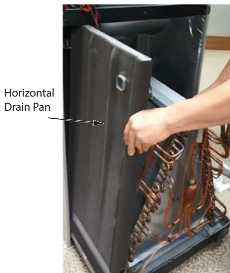
Figure 18: Evaporator Coil/ Drain Pan Assembly.
