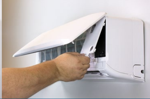
Remove electrical access panels (2)
