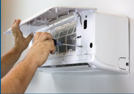
Back out electrical panel screws
