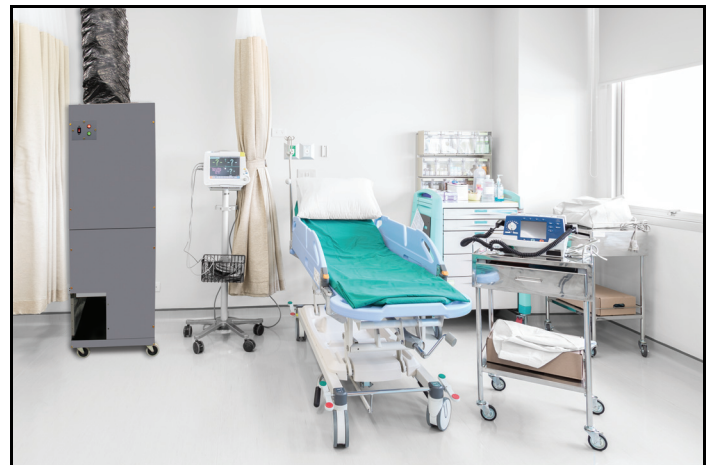
Fig. 2 – Room Setup Example for Negative Air
