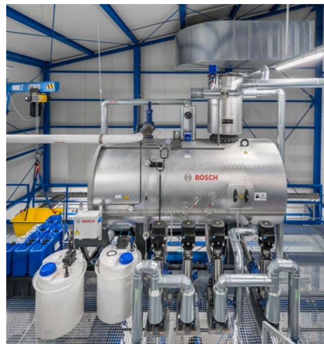
Water service module WSM
