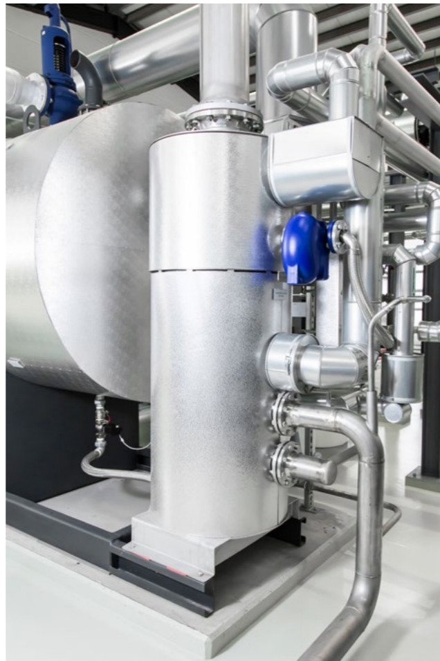
Expansion, heat recovery and blow-down module EHB
