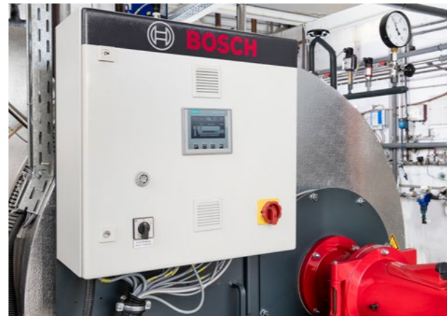
Compact steam boiler control CSC
