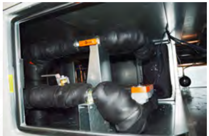
Refrigerant-to-Water Heat Exchanger with fully modulating water control valve. ▶
