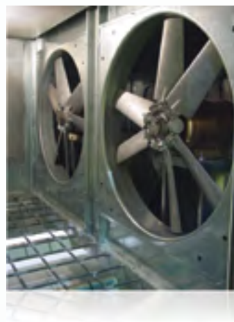
◀ Direct Drive Axial Flow Exhaust/Return Fans are more energy efficient and require less maintenance than belt driven fans.
