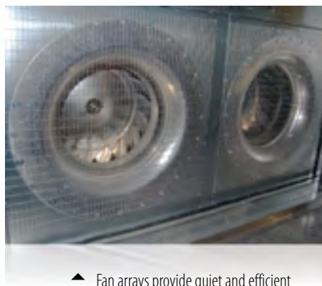
▲ Fan arrays provide quiet and efficient airflow through multiple fans.
