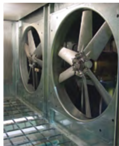
▲ Direct Drive Axial Flow Exhaust/Return Fans are more energy efficient and require less maintenance than belt driven fans.
