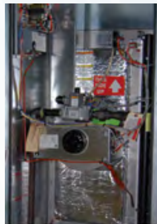
▲ Factory installed indirect fired gas heater provides energy efficient heating.
